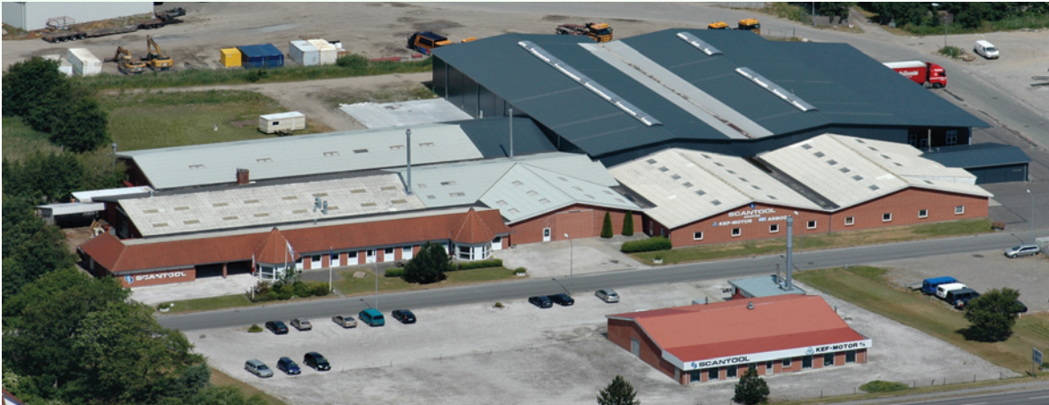
The Factory in Brovst Denmark
